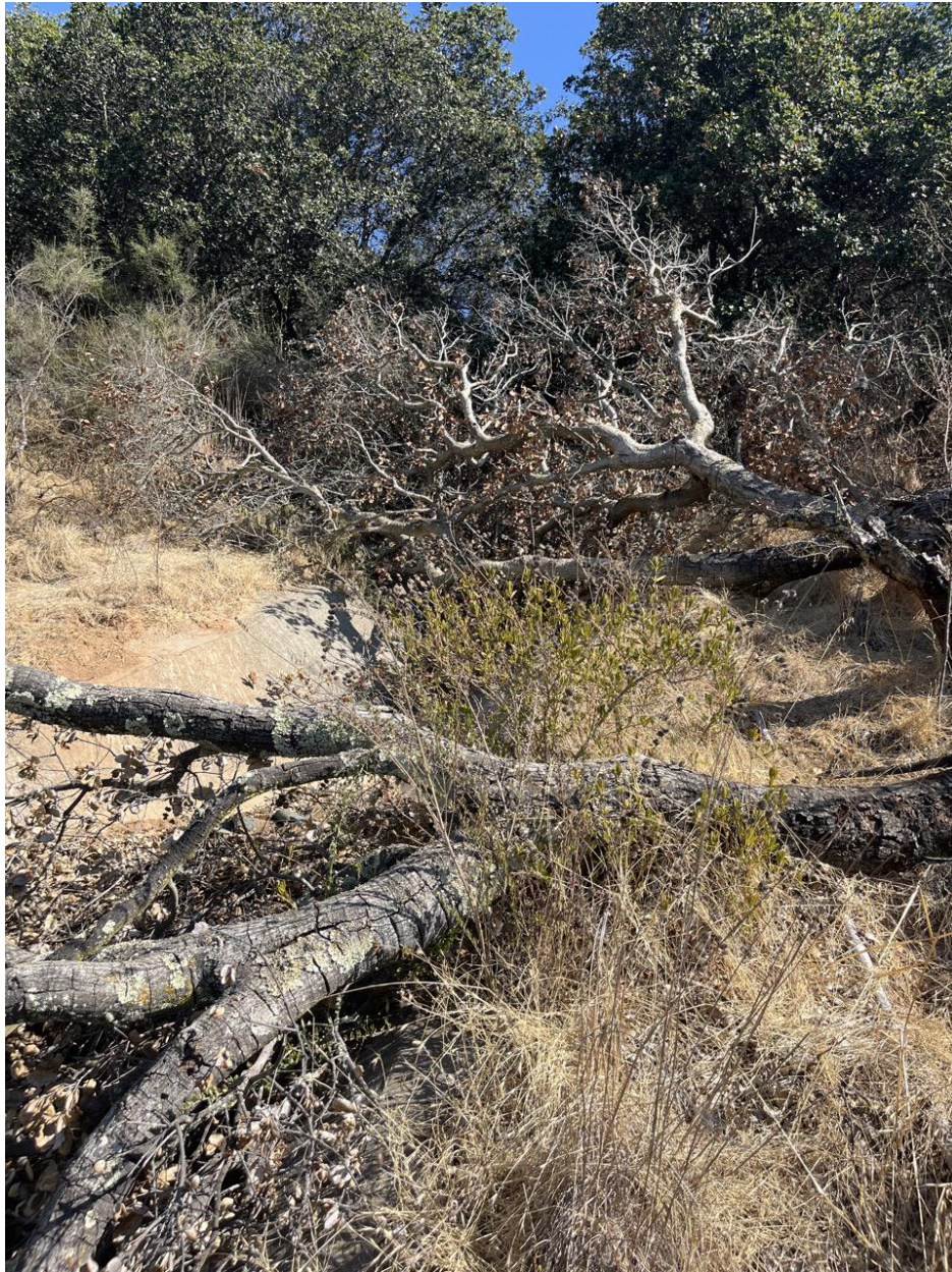
Fallen tree and leaves from oversteepened slope deposited in the concrete-lined drainage ditch on Parcel F
