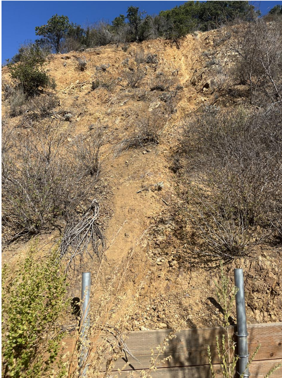
Erosion gully formed above drainage ditch and wood-lagging debris wall, eroded material deposited behind wall and in drainage ditch.
