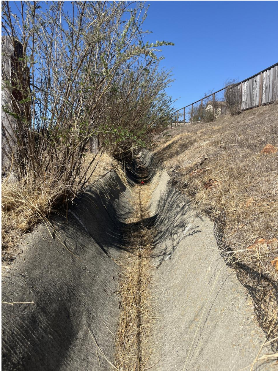
Overgrown vegetation within 6 inches of concrete-lined ditch.
