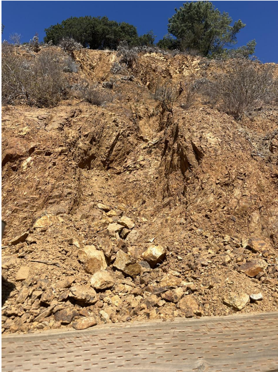
Raveling and eroded material filled debris wall up to capacity
