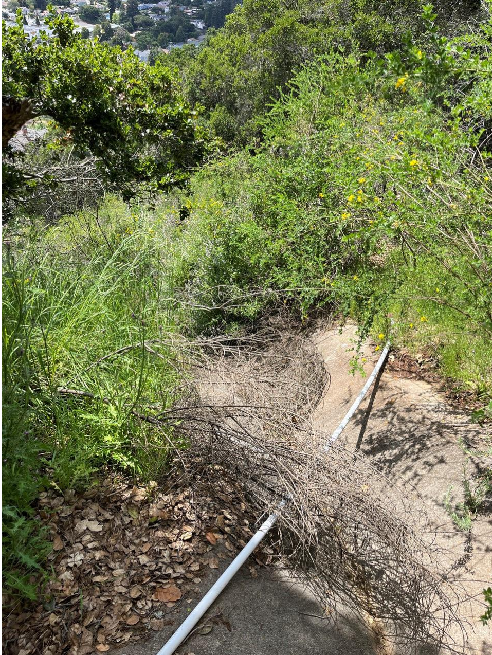
Fallen tree and leaves from oversteepened slope deposited in the concrete-lined drainage ditch on Parcel F
